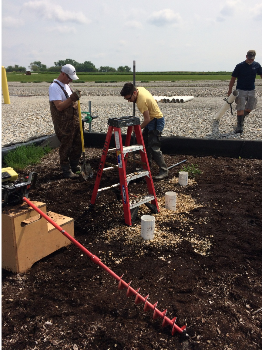
Figure B.2 Modified ice auger used to drill the monitoring wells in the SAGR.
