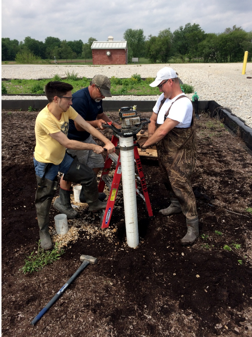
Figure B.3 Process used to drill monitoring wells in the SAGR.
